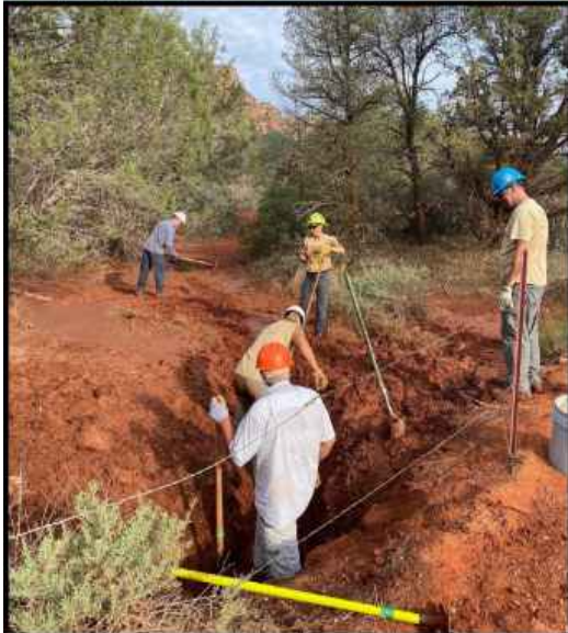
The crew clearing the drain and a new channel on Bell Rock Pathway.
