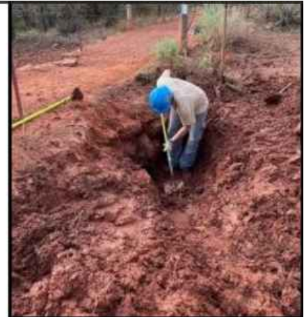
The crew clearing the drain and a new channel on Bell Rock Pathway.
